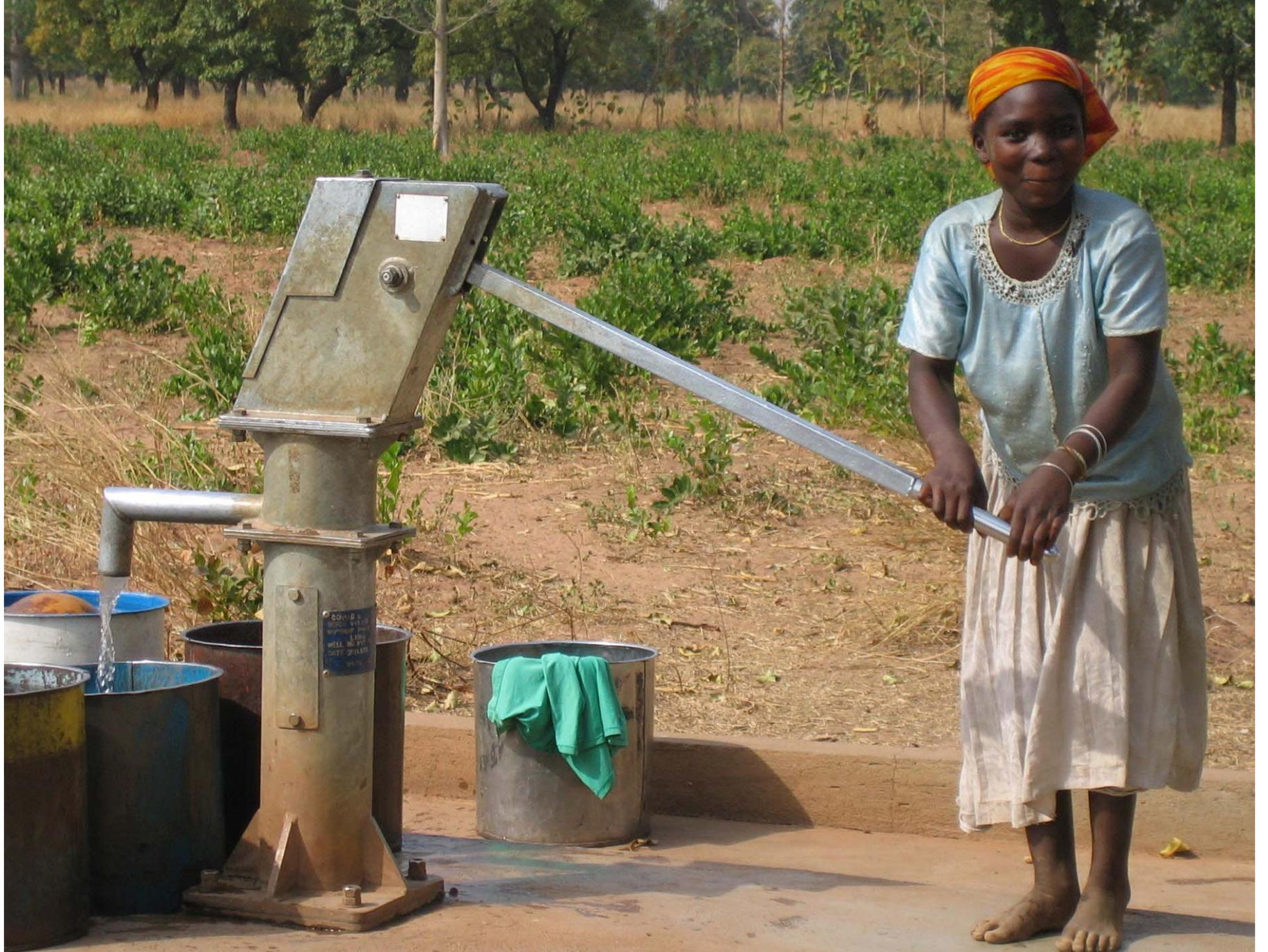
**Deep Borehole Well with Lift Pump**
