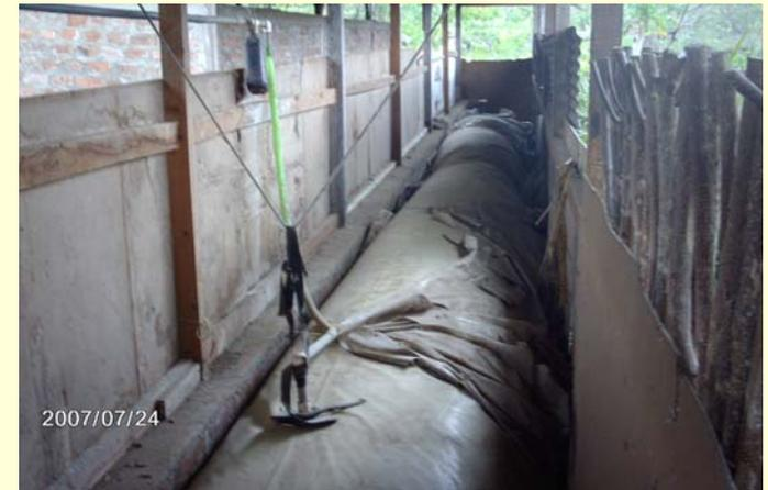
Current biogas technologies use a single low density plastic liner (such as a low grade polyethylene) as the container for a plug flow digester system. The system is inexpensive, but **vastly inefficient** and problematic. Various problems including frequent **breaks and leaks** (as seen in the image to the left), and a **high residence time** (defined as the time it takes to yield biogas output from a biomass input), consistently retard production of biogas.
