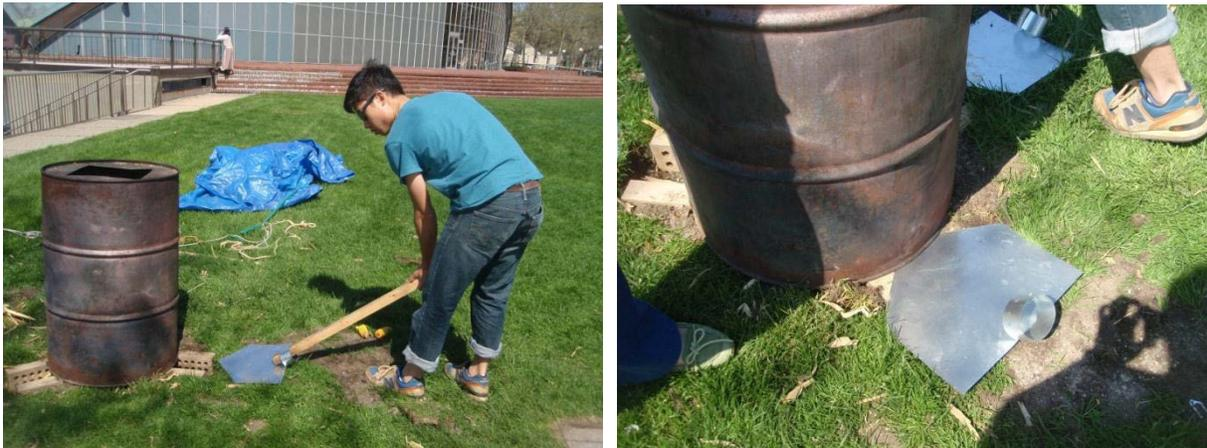
**Figure 12** – Metal seals inserted between bricks/ground and the barrel
