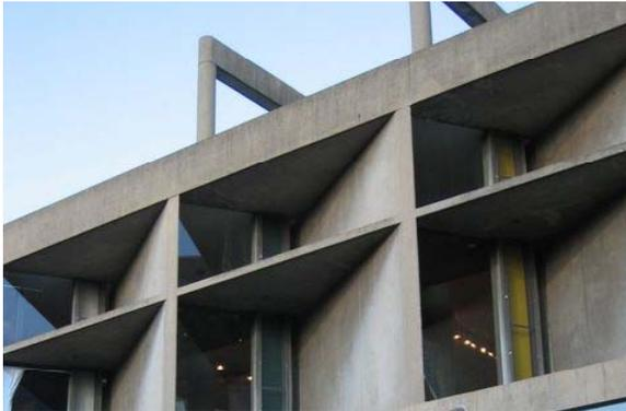
The opaque *aerateurs* and the protruding layer of concrete that juts out between each window make the shading system for the south façade. The north façade does not have a specific shading system but is shaded by the other floors above it and the building on the other side of the ramp.
